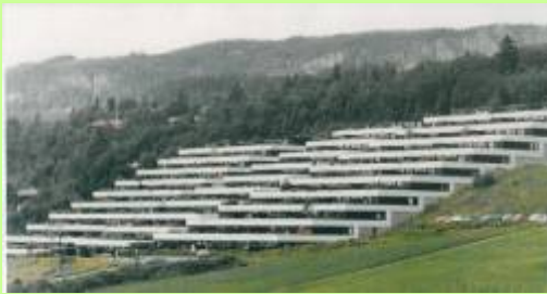
Original facades from 1970
